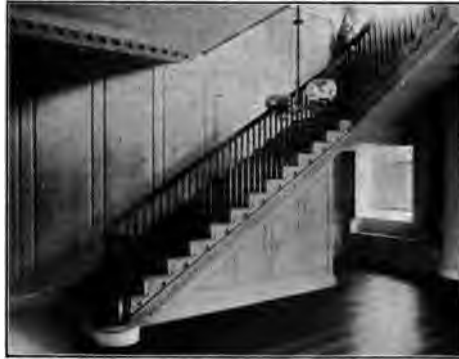
Staircase, Carvel House
